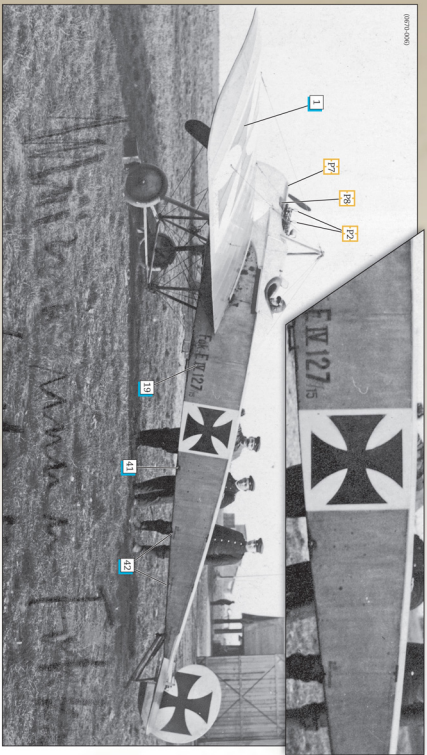
This photo of Max Immelman seated in his Fokker E.IV 127/15 appears to have been taken on the same day as the photo opposite. Note the uneven finish of the fuselage fabric. Bloody castor oil stains soaked through from the inside and the struts above the bottom longeron. Despite having been extensively damaged on 31 May (see page 22), 127/15 was reportedly back in service in time to be damaged again 18 June 1916, forcing Immelman to use Fokker E.III 246/16 that evening when the Fokker pilots of Keel Doan intercepted 7 FE.2b of 25 Sqn. After joining in the dogfight it appears that, during combat with FE.2b 4909 (see Wingnut Wings model 3201-4 FE.2b Early), the MG synchronization gear failed and he shot off his own propeller. The resulting violent vibrations caused his aircraft to shake itself apart and Max plummeted to his death 2000 meters below. It is widely recounted that Immelman shot down 2 FE.2b on this day but these were not officially recognized, so his total victory count remained 15. He was 26 years old.
